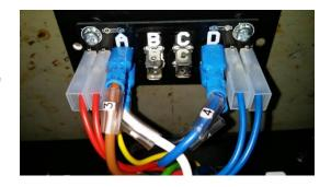
Connect cable "5" to one of the spade lugs labelled "B" Connect cable "6" to one of the spade lugs labelled "C"
