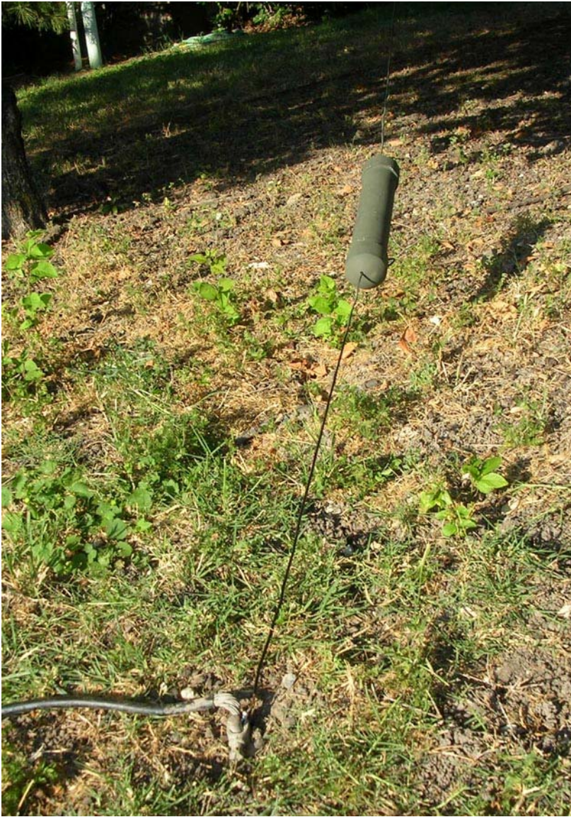
A permanent termination of the load to a ground rod system, ground wire is clamped to several rods. Notice the Termination floats with the cooling / weep holes down
