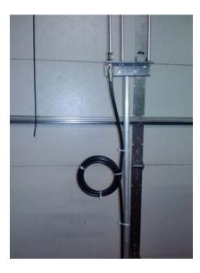
Lastly, grounding the antenna is not necessary for performance. But, it can be grounded for lightning protection by grounding the assembly bracket. This will not affect performance.
