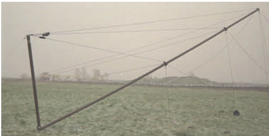
Tilting of a 15m mast
