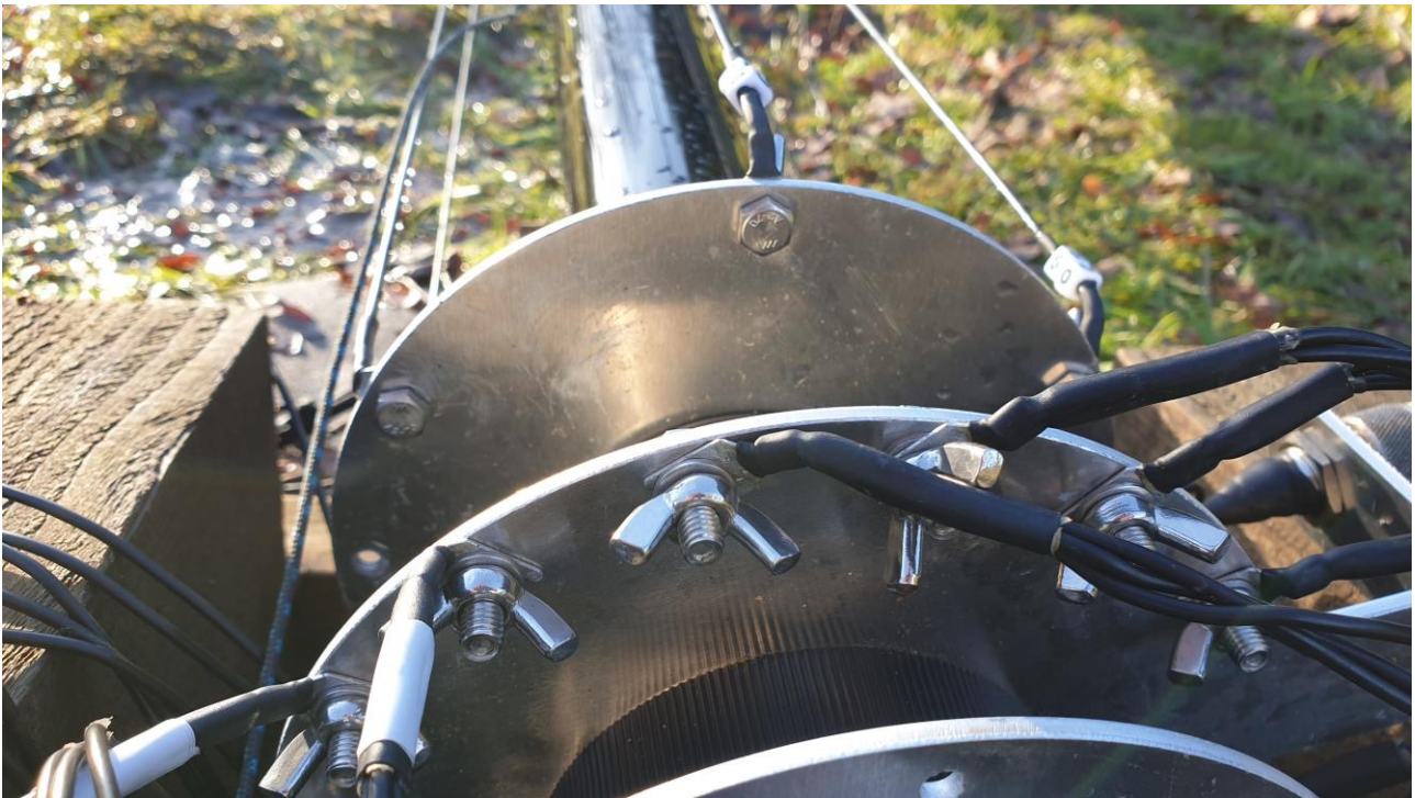
Looking up the pole from base. Note how fork connectors are sealed from the weather with small sections of heat-shrink. Ignore the white tape on the radials – these were indicators for me that these radials were shorter. 80m and 60m elements are on the left and right of driven plate so that they match the curve of the pole during construction..
