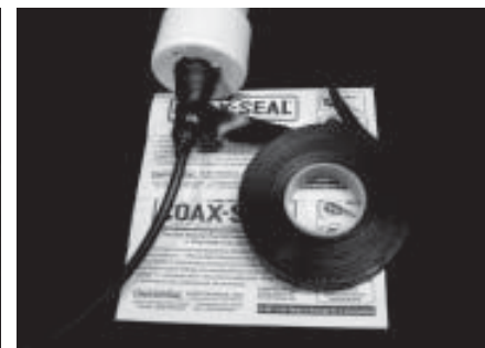
Optional, but recommended, apply a layer of Cold-shrink tape completely over the Coax Seal.
