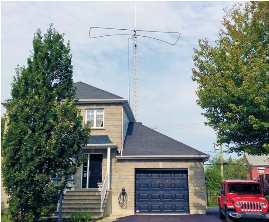
Figure 8 — The UrbanBeam installed on the author's tower on his small lot. An inverted V for 80 meters hangs just below the beam.
