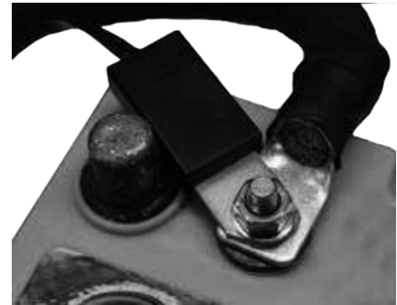
Fig 2.5(b) Temperature Sensor Installation
