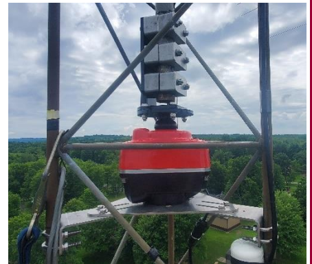
Install at K3LR with DXE-SDMC-2HD
