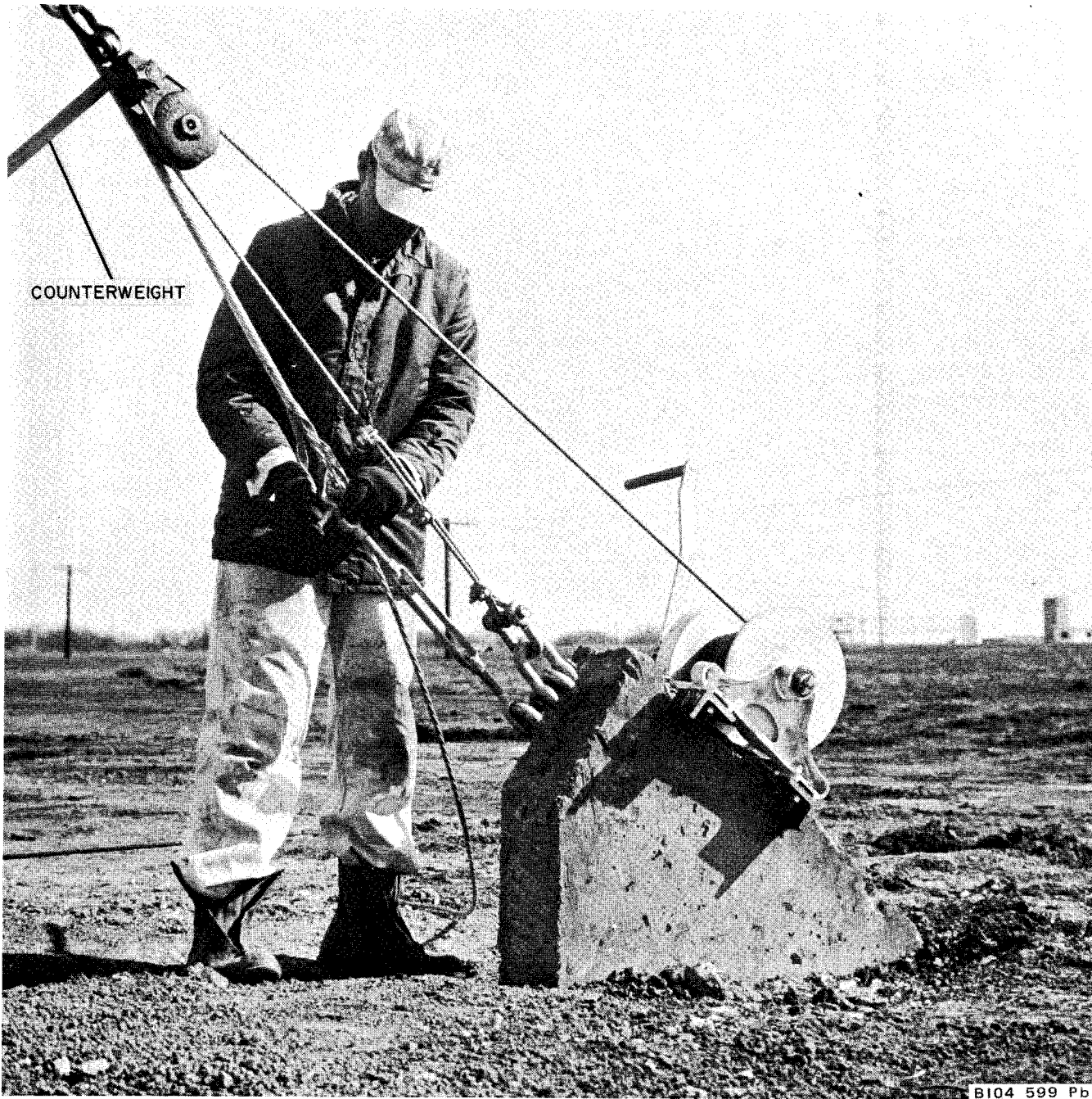
Figure 2-14. Winch and Block Assembly in Use.
