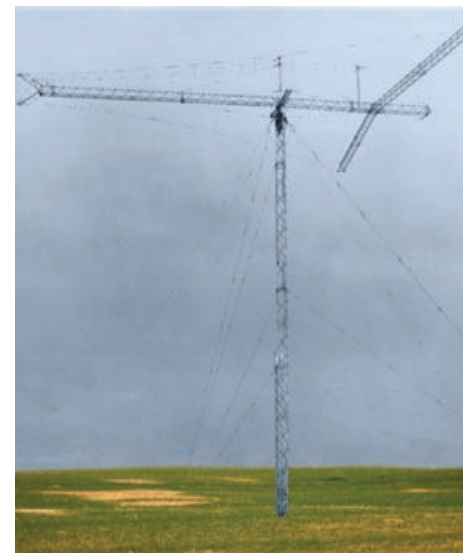
The TCI Model 521—a compact, easily erected antenna that has been providing highly reliable service since it was introduced in 1973.
