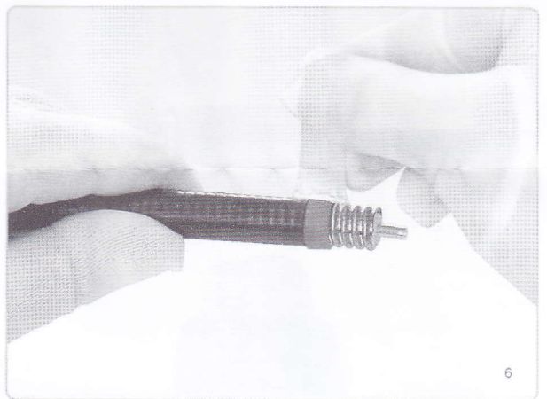
套上密封圈并涂上油脂 Put the gasket onto the cable and then wipe the gasket with the grease.
