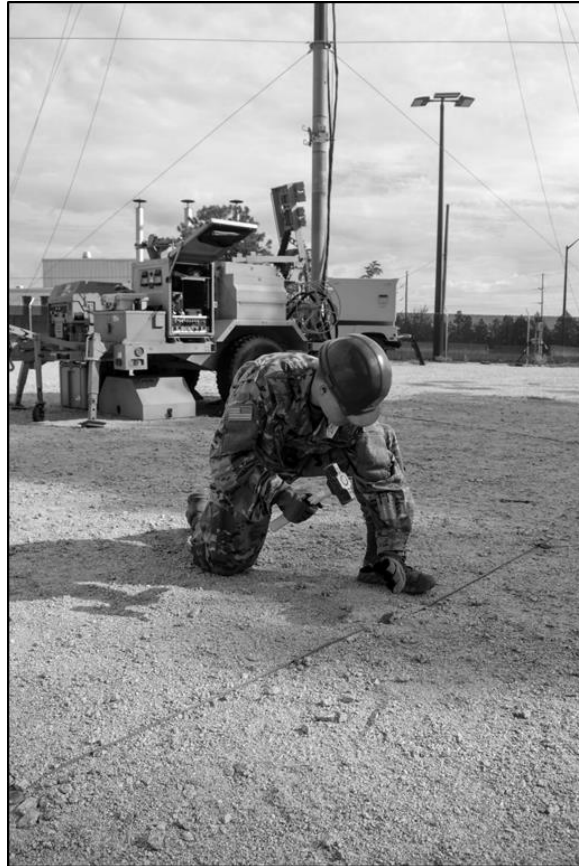
Figure 2-10. Surface wire grounding kit installation
