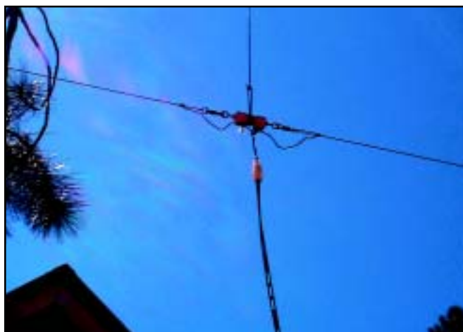
The feedpoint of the 160 meter horizontal loop mounted about 15 feet above ground. The photo shows the twin-lead feed line and support rope. The center insulator was made using PVC pipe, end caps and screw-eyes.
